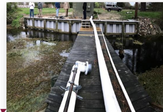
Hampton Roads Bulkhead Replacement
