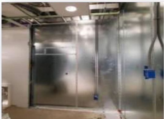
Roanoke Riverside 4 MRI Shielding Installation
