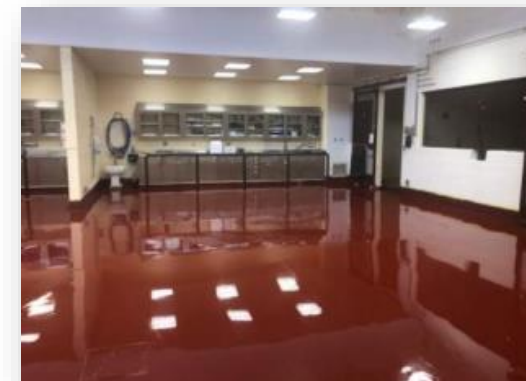
Equine Medical Center New Treatment Floor
